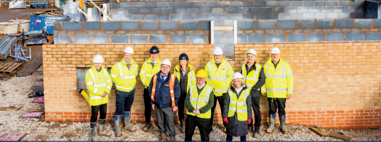
70 new homes are being built on the Whiteleas Avenue site at North Wingfield Progress visit to site included Rykneld Homes staff, Countryside Partnership staff and Cllr Nigel Barker
