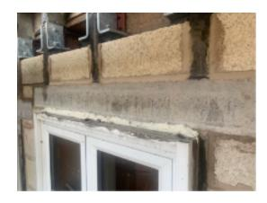
Your new upvc ground floor double glazed windows will be fitted. These are fitted externally and any making good and sealing with be carried out inside your home.
