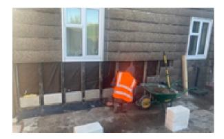
Works will commence with the first rows of panels being removed. The pictures show the structural block-work in progress.
